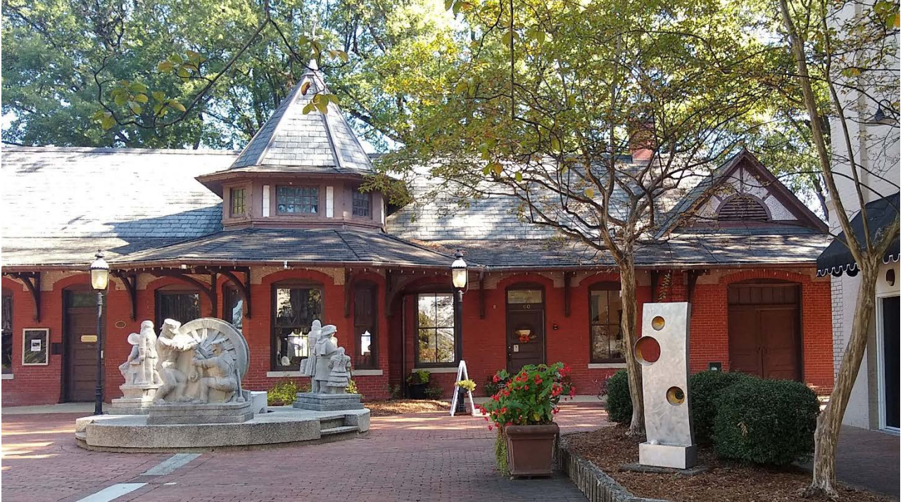
Figure 13 Southern Railway Passenger Station in Downtown Burlington
