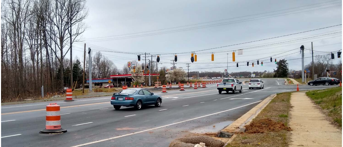
Figure 57 Roadway Improvements under Construction in Mebane
