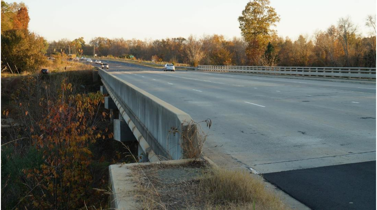
Figure 22 NC 54 Bridge over the Haw River
